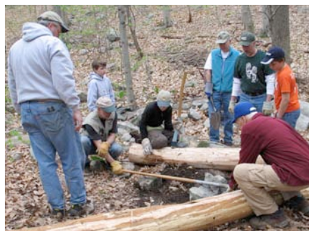
Bridge work - photo by Terri Peters
